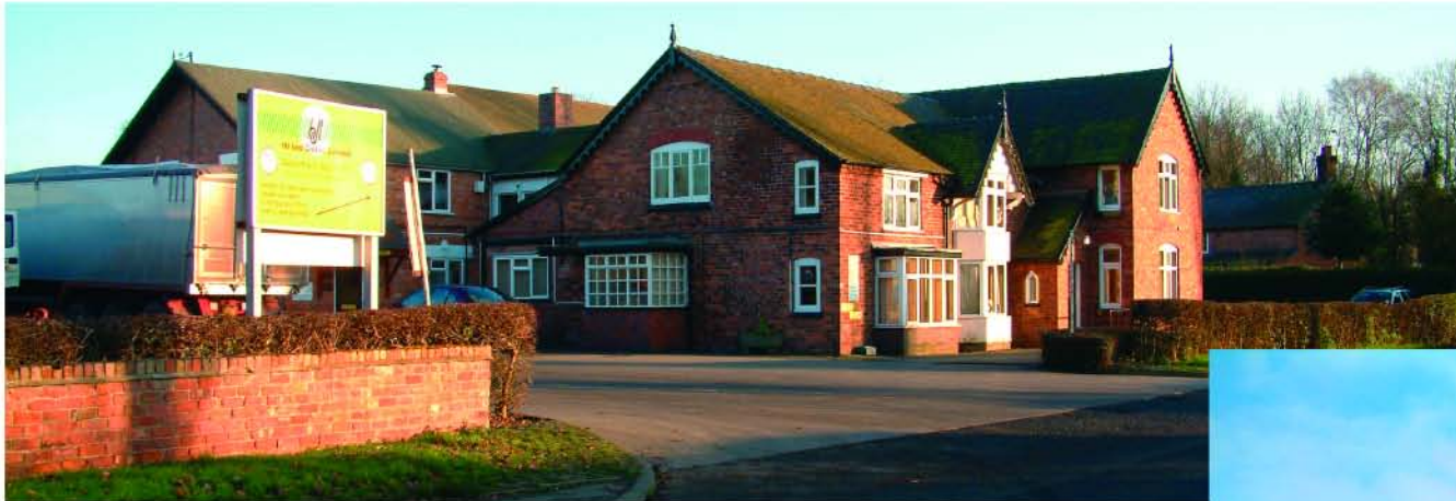
Aston Mill entrance
